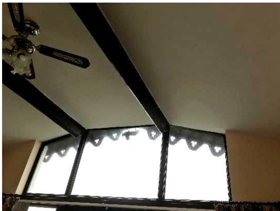
Plate 8 – Internal character of the second-storey of the extension
