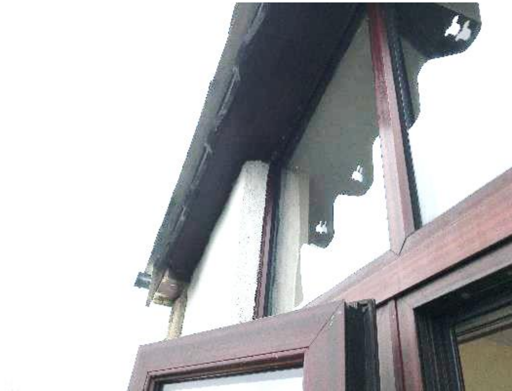
Plate 9 – Underside of the eaves viewed from the balcony
