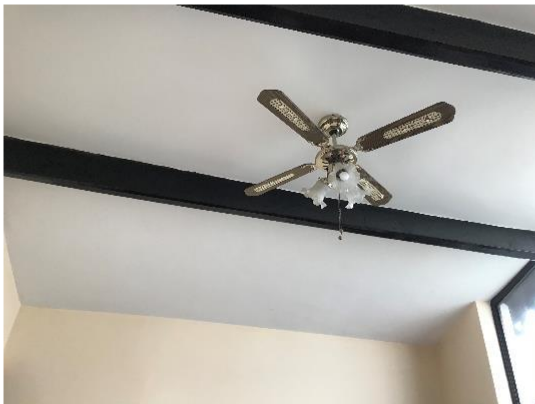
Plate 7 – Internal character of the second-storey of the extension
