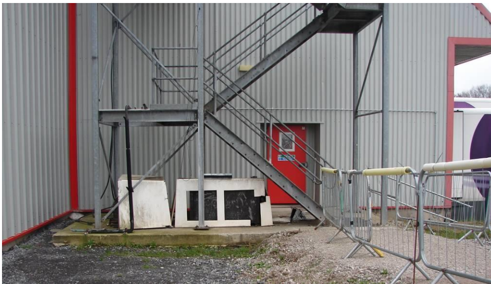
Example of the concrete plinth and paving slabs associated with the fire escapes.
