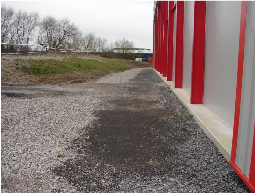
A view of the western elevation of the existing building.
