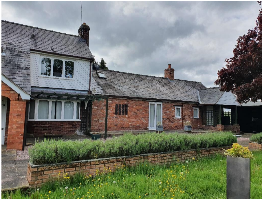
Photo of side elevation part 2
