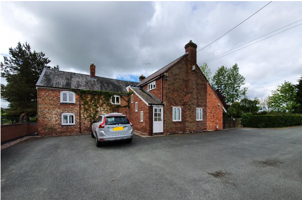
Photo of Front Elevation taken from main road side
