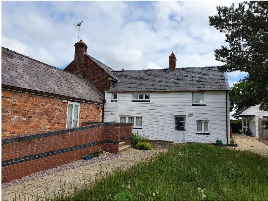
Photo of Rear Elevation
