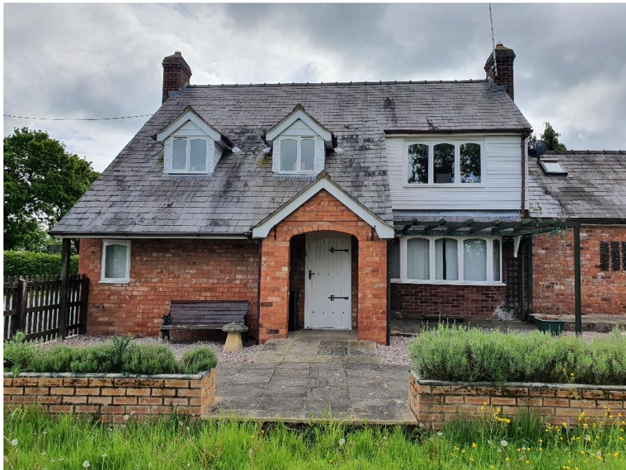
Photo of side elevation part 1
