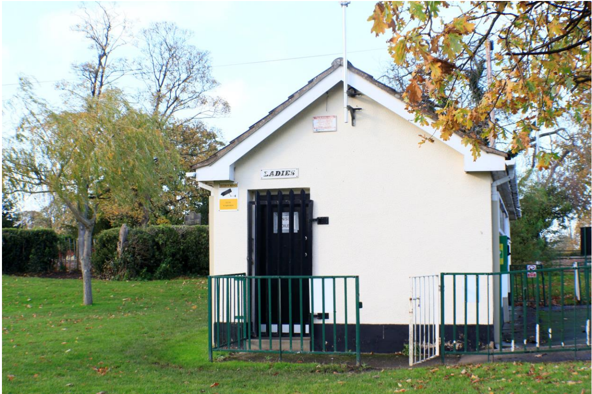
End elevation from park
