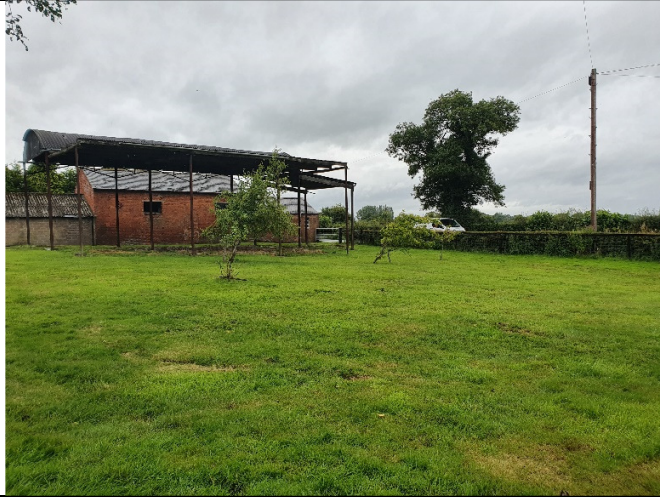
OVERALL VIEW OF SITE FROM EAST
