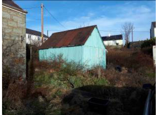
12.01.18 – Outbuilding directly adjacent to west of site; constructed from corrugated metal.
