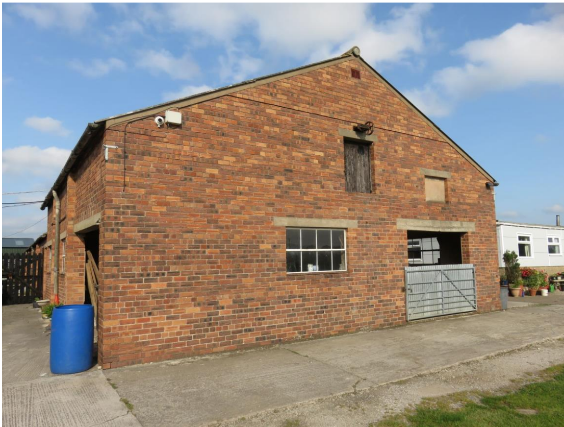
Photograph 2 – Eastern aspect of barn
