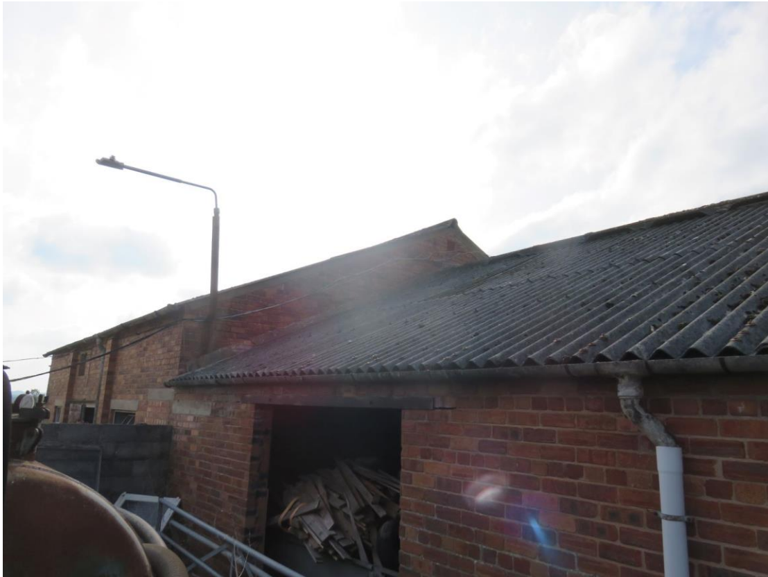
Photograph 5 – Western aspect of barn viewed from northwest
