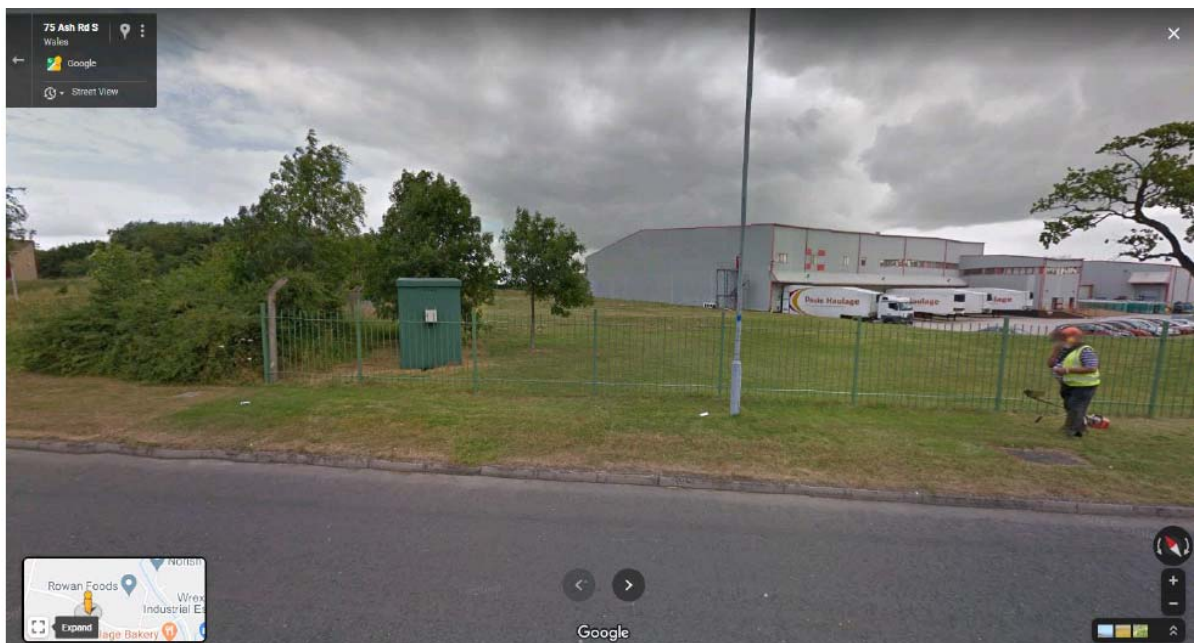
Photos of application site
