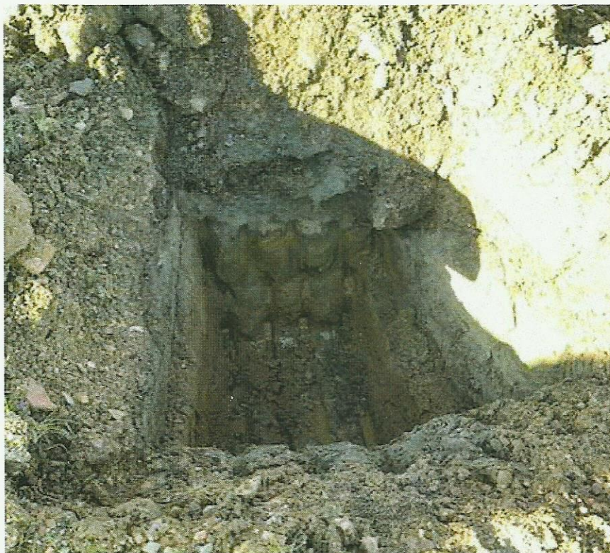
TP04- Pit Walls
