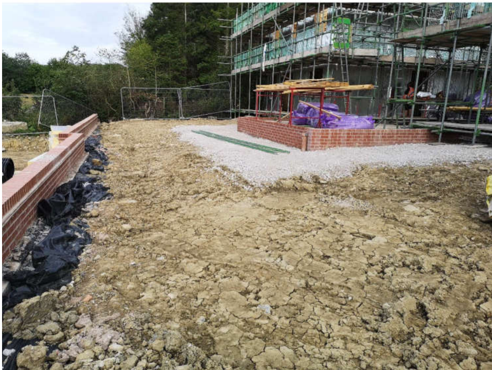
Exposed till fill behind retaining wall at Plots 5/6
