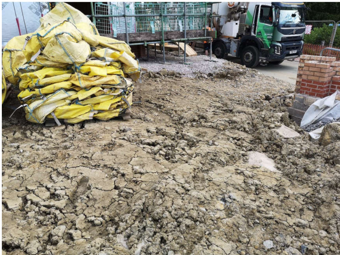
Exposed till to front of Plot 4, showing access road
