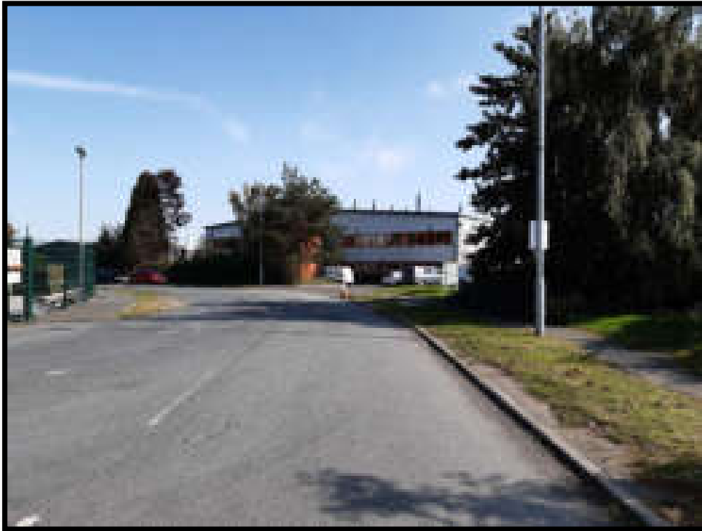
Photograph 3. Looking east at existing Magellan building.
