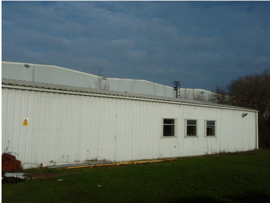
Building at Target Note 1a ; eastern side.
