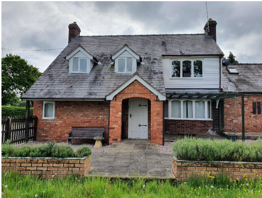
Photo of side elevation part 1
