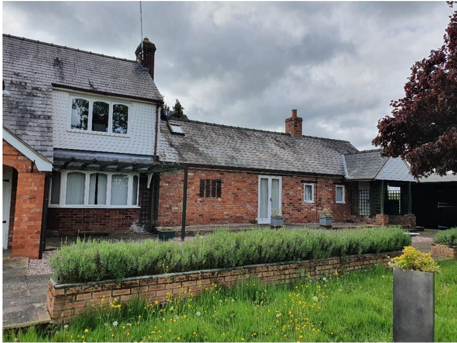
Photo of side elevation part 2
