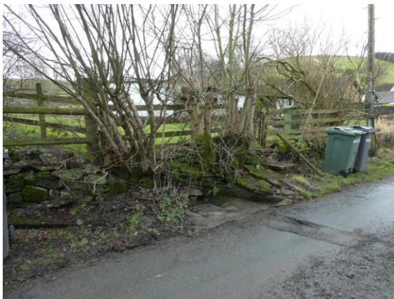
Photo 6: north boundary (laneside) of NE corner
