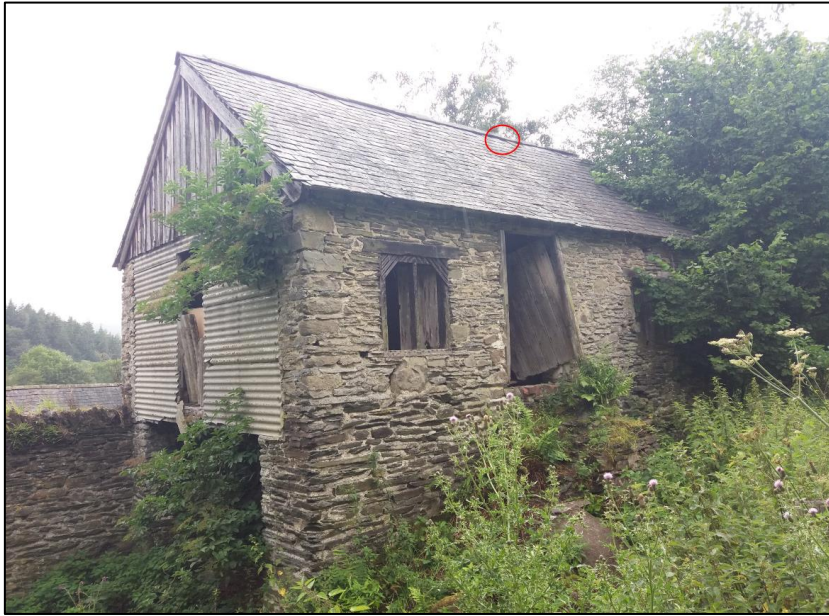
Another soprano pipistrelle was observed entering B2 at the apex of the eastern gable end (circled in red below).
