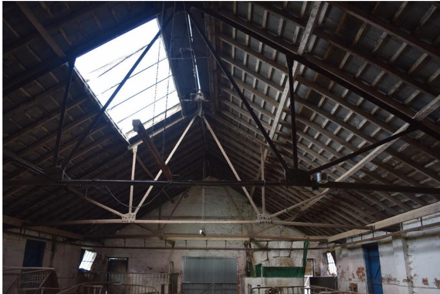
Figure 4.8. Roof space of building 2
