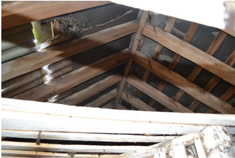
Figure 4.12. Roof space of building 3
