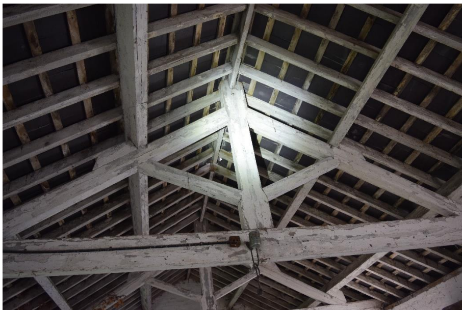
Figure 4.3. Roof space of building 1
