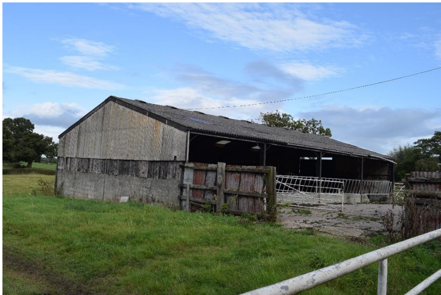
Figure 4.15. External view of building 4 from southwest
