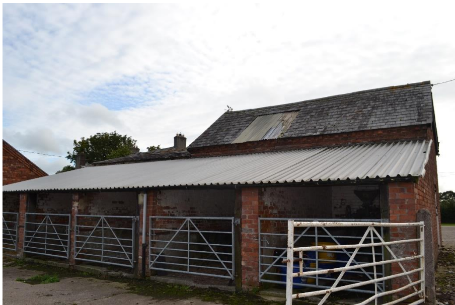
Figure 4.11. External view of building 3 from north
