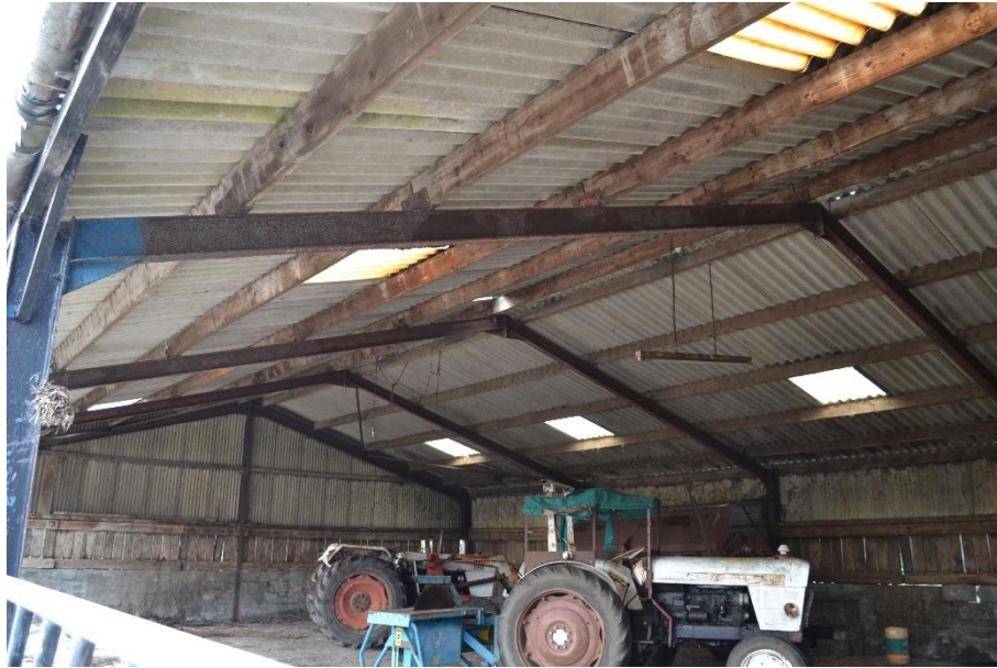
Figure 4.16. Interior of building 4
