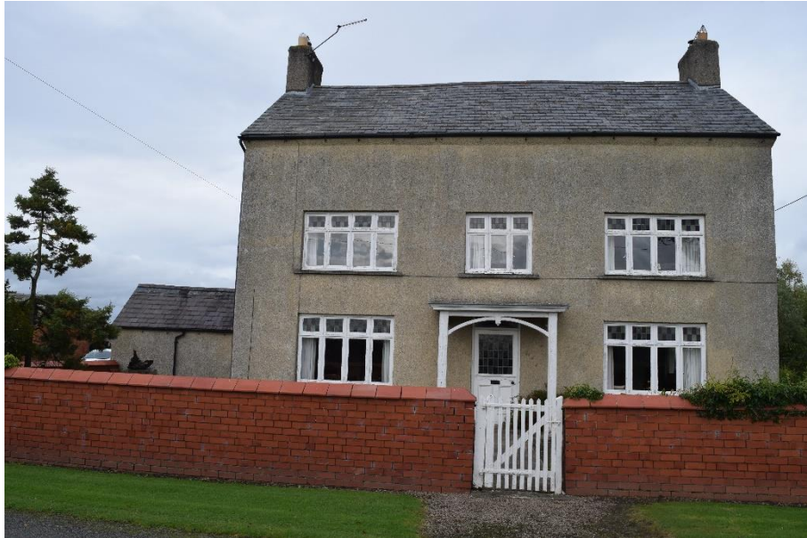
Figure 4.20. Farmhouse to east
