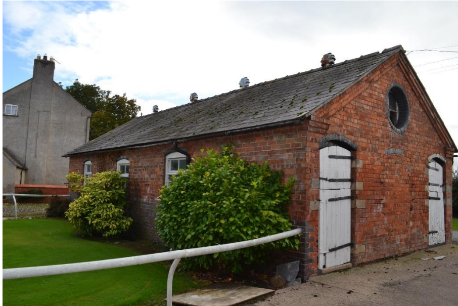
Figure 4.2. External view of building 1 from northwest
