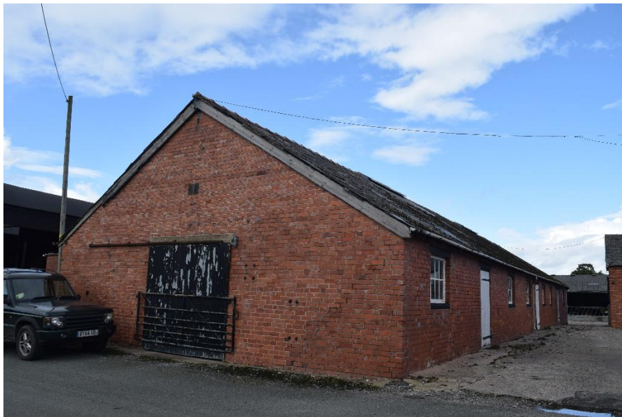
Figure 4.7. External view of building 2 from south
