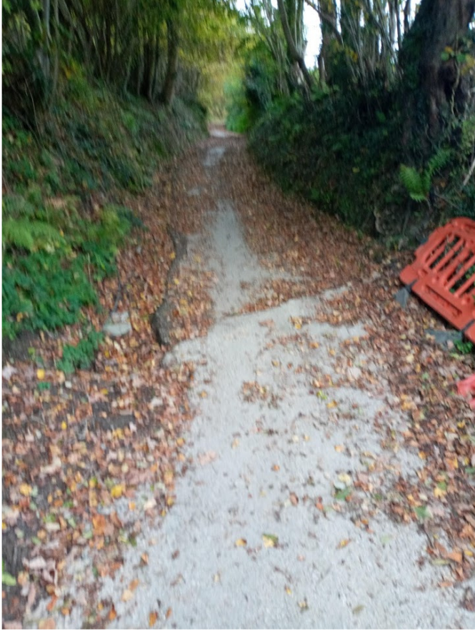
Existing road with narrow width and steep, dense embankments
