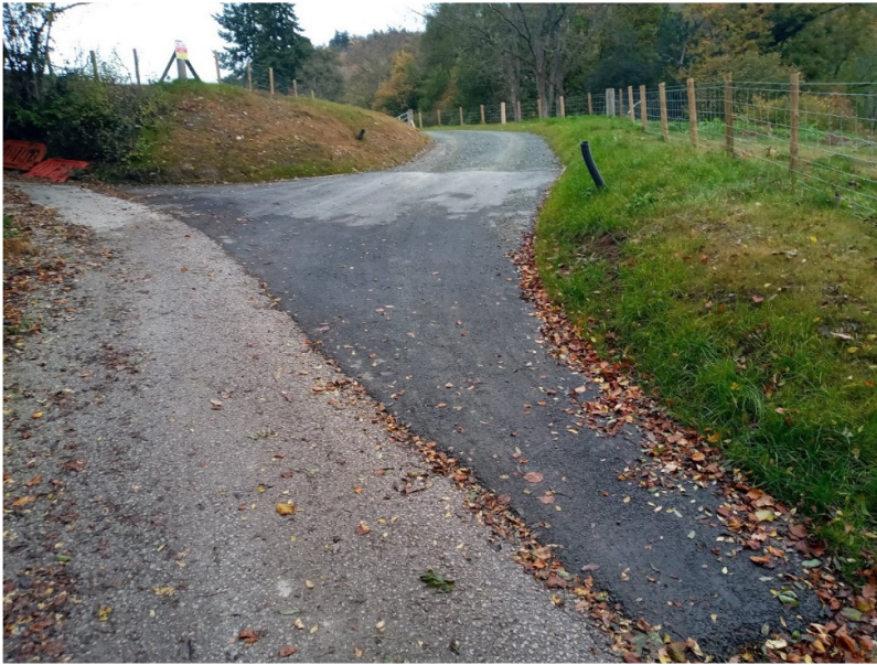
Access drive entrance off existing road
