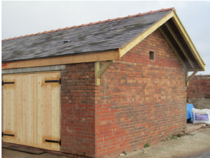
Photo 4: Open ‘fly-in’ access provided in South gable-end.
