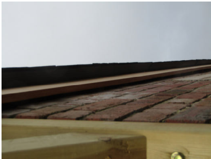
Photo 5: Gaps left between wall and eaves for access for crevice-dwelling bat species.
