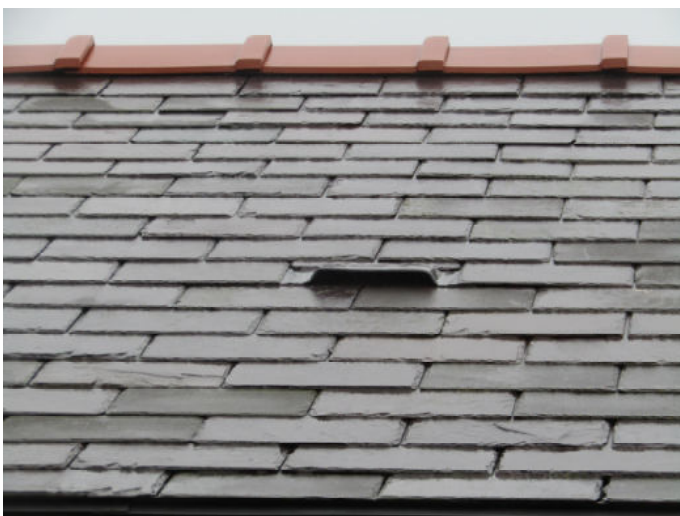
Photo 3: Bat slate installed into slate roof.
