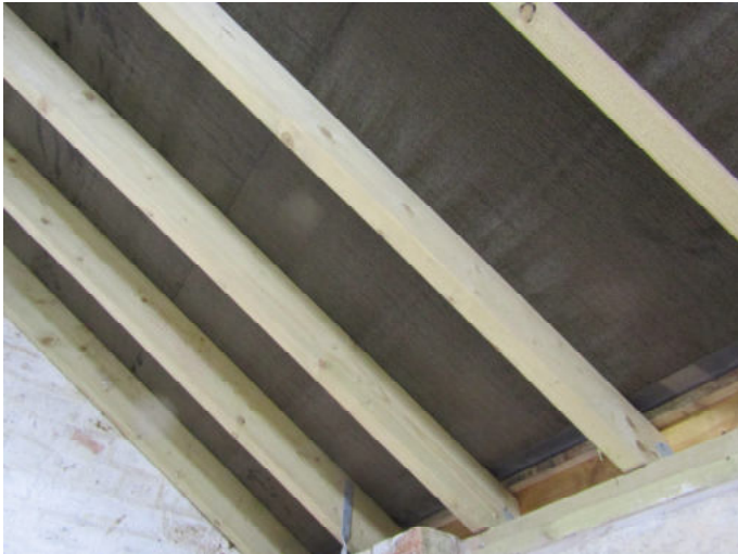
Photo 1: 1F bitumastic felt used beneath slates in new bat loft.
