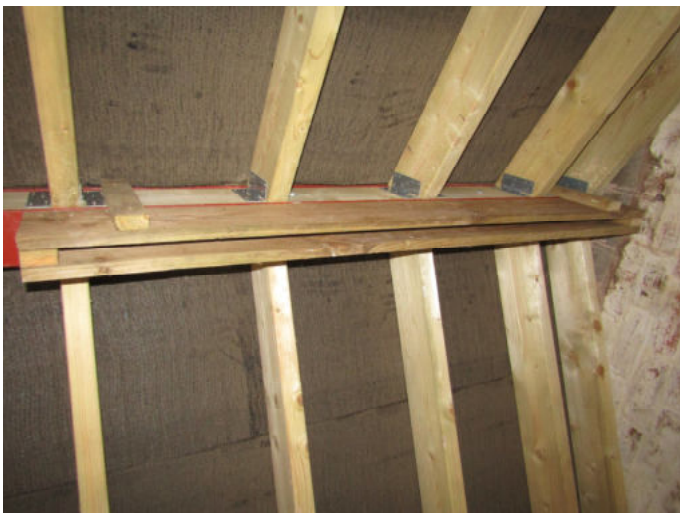
Photo 2: Crevice boxes have been installed in the new bat loft.
