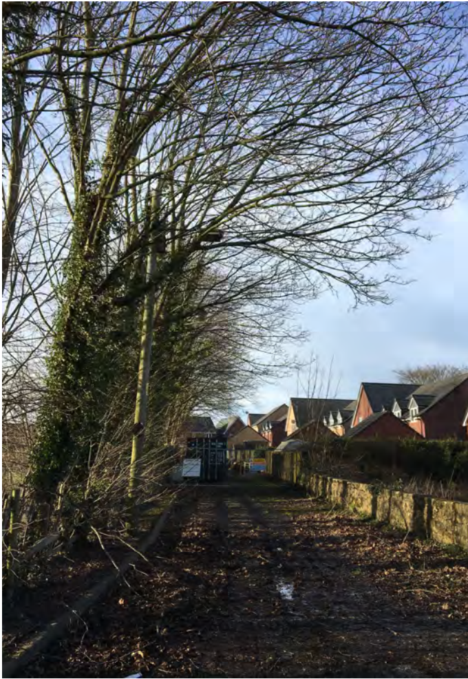
G1 & existing highway surfacing
