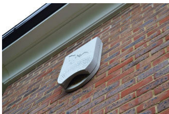
Figure 11: Schwegler (1WQ) bat box fitted to wall.
