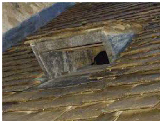
Figure 17: Lesser Horseshoe covered porch entrance.
