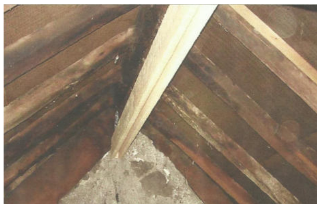
Figure 20: Crevice box in loft void.
