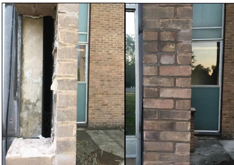
Figure 3: PRF identified during the preliminary roost assessment (Left) and during the dusk emergence survey (Right).
