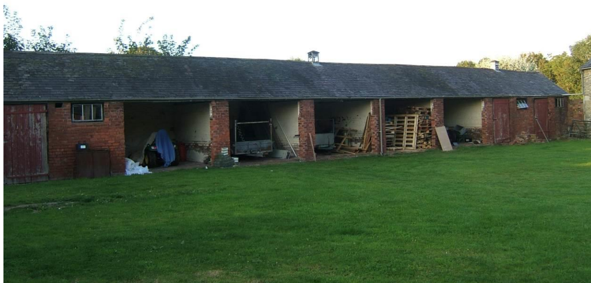
Figure 1: South elevation of Building 1.
