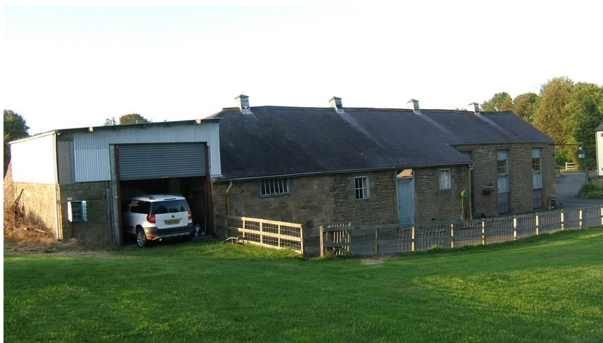
Figure 7: South elevation of Building 3.
