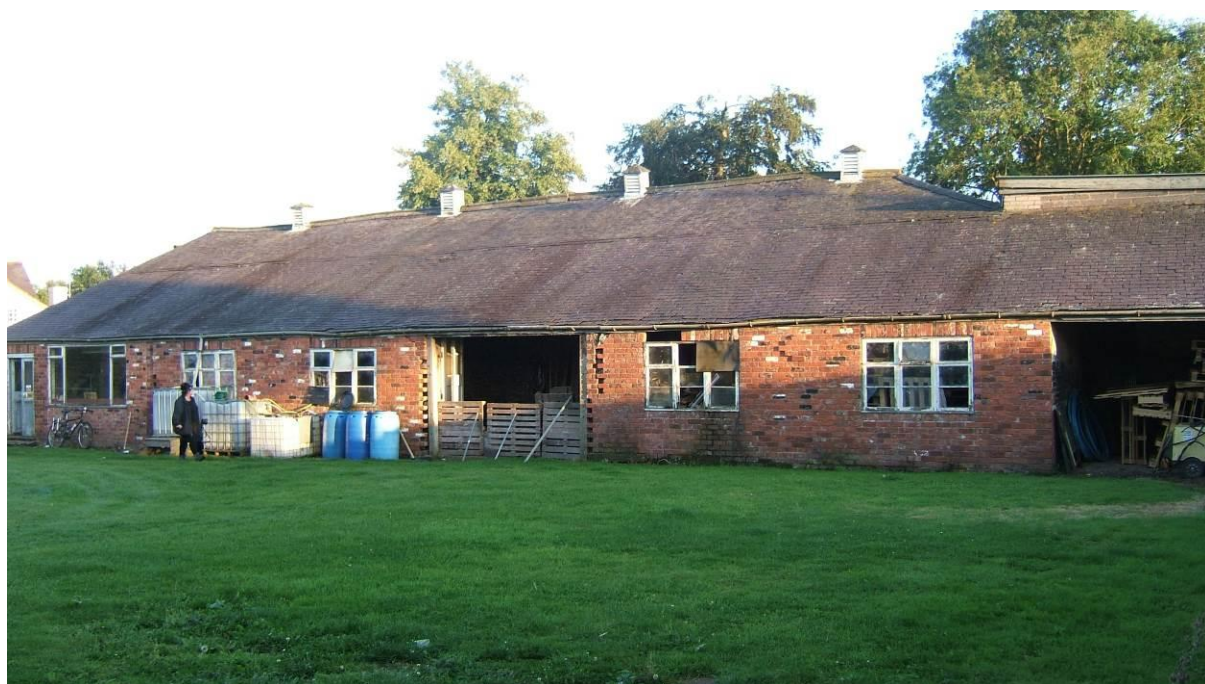
Figure 6: North elevation of Building 3.
