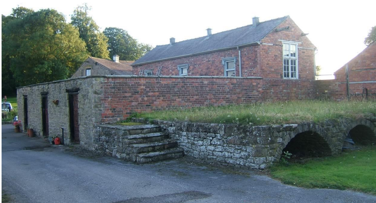
Figure 3: Northern gable of Building 2.
