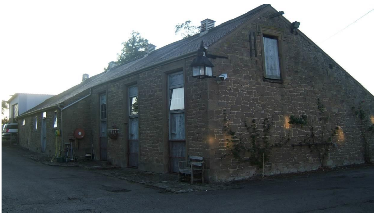
Figure 8: Eastern gable of Building 3.
