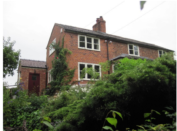
Existing house from site of new garage
