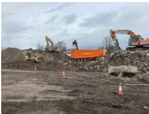
Photo 1: View eastwards across the site on 4th December 2020, with the former position of the tank being located underneath the demolition material stockpile on the right (as indicated by Braithwaites). A stockpile of crushed material is present to the left of the orange metal skip in the background.
