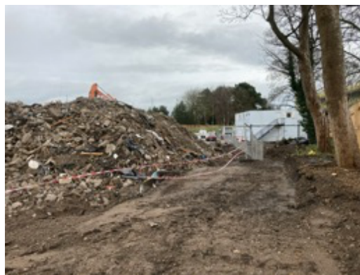
Photo 2: View southwards across the site on 4th December 2020, with the former position of the tank being located in the left foreground.
