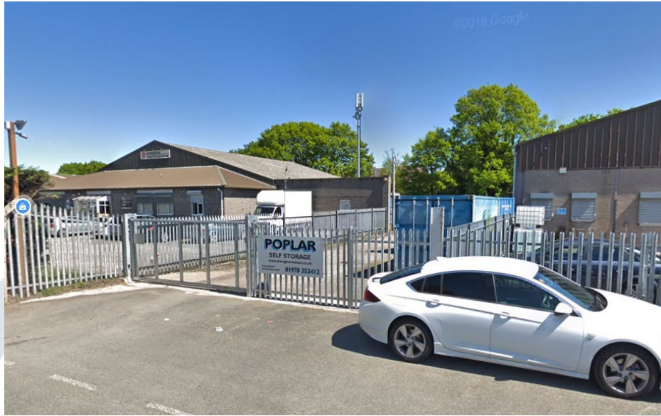
Figure 2. View of existing mast to the rear of Howden's commercial building from Industrial Main Road (ground level radio equipment housing and apparatus in secure compound not shown) taken from Google Streetview.
