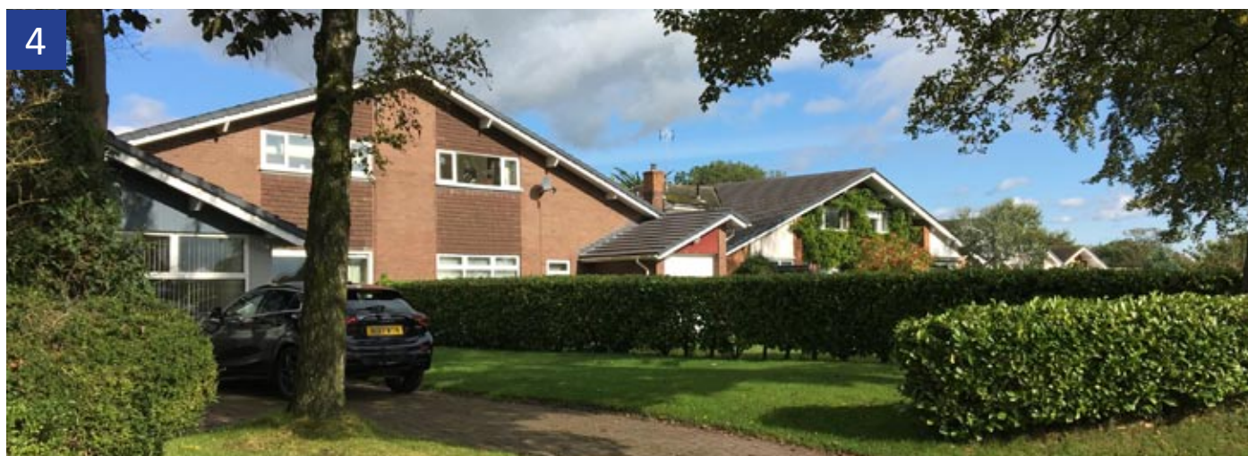
Photo looking north-east along Hillock Lane of 2 storey semi-detached properties set back from a narrow country road by large front gardens with hedging.
