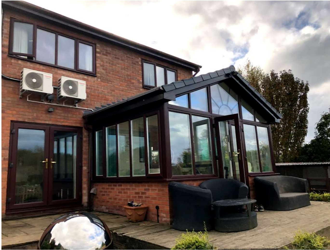
Existing rear elevation, showing conservatory to be replaced.
