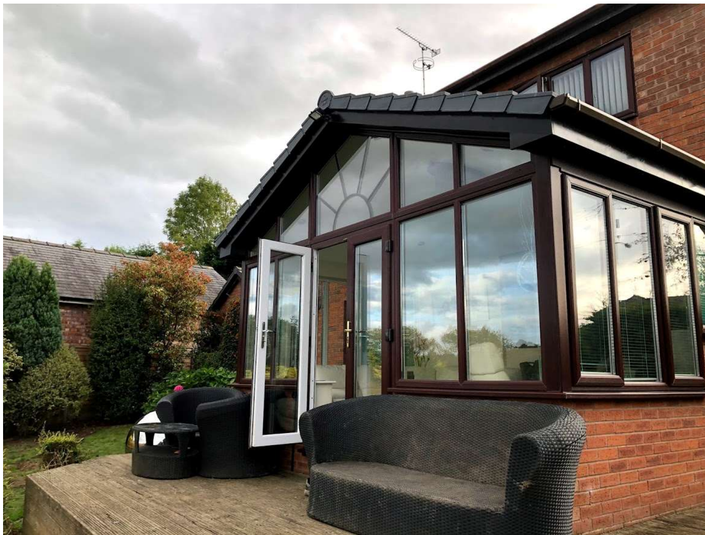
Existing rear elevation, with views to neighbouring property
