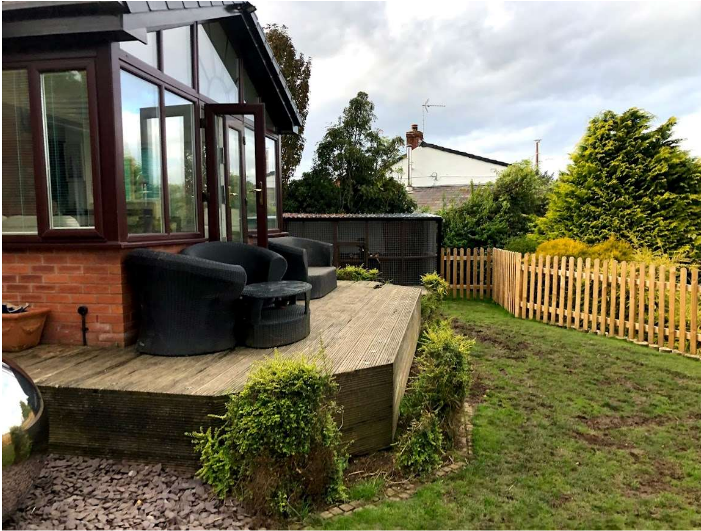
Existing rear elevation, with views to neighbouring property
