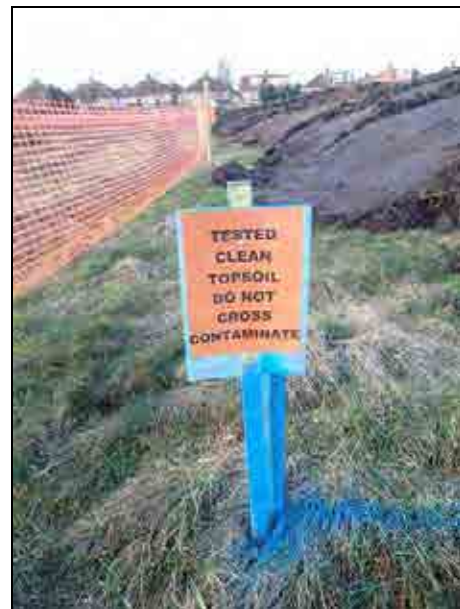
Photograph 15: Example of good stockpile management with warning signs and fencing to prevent accidental cross-mixing.
