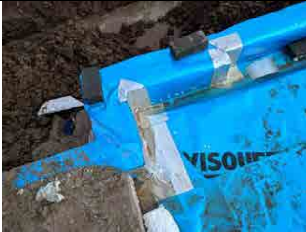
Photographs 8 and 9: Formed corner sections correctly taped
