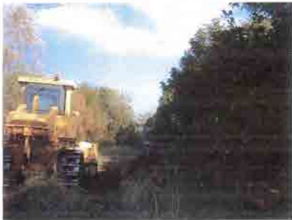
Stripping of topsoil to create reclamation site access road (2003)
