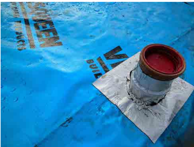
Photograph 4 and 5: Check top hat is sealed to membrane and pipework with tapes, and Jubilee clip, or detail strip installation.
