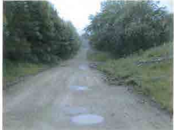
Cycleway along northwestern strip following placement of topsoils along western edge to narrow road (May 2007)
