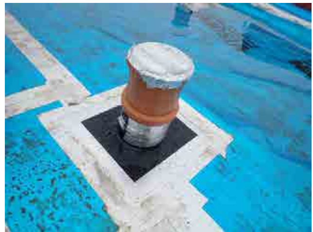
Photograph 4 and 5: Check top hat is sealed to membrane and pipework with tapes, and Jubilee clip, or detail strip installation.
