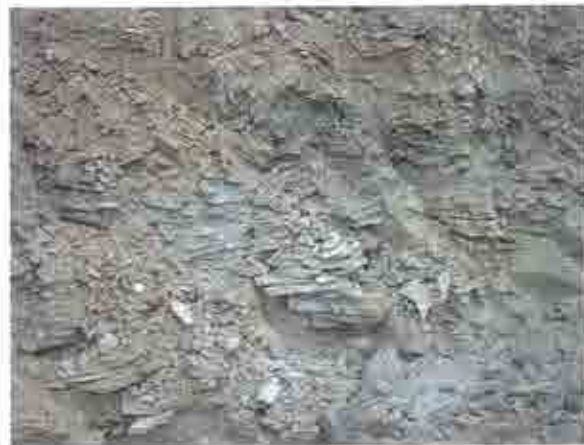
Typical sandstones encountered within LRDM during excavation and replacement activities
