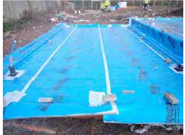
Photograph 2 and 3: Check general condition of gas membranes with photographs showing the plot in context.
