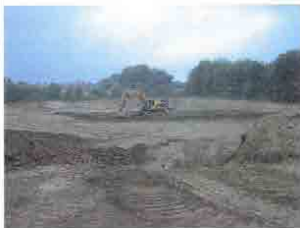
On-going re-compaction of materials in LRDM (July – October 2007)
