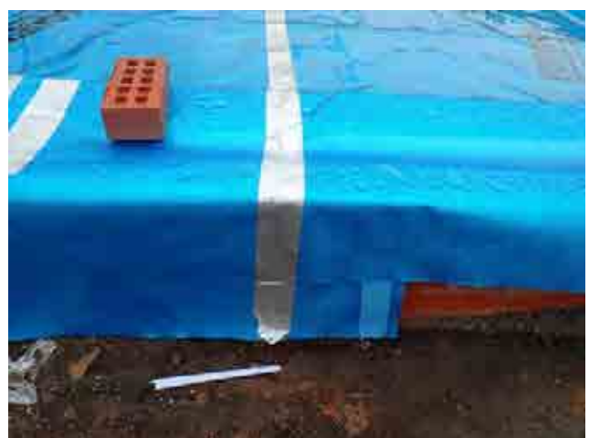
Photograph 6 and 7: Check >150mm overlaps of membranes and proprietary tapes placed and sealed or heat welded jointing with photographs taken.
