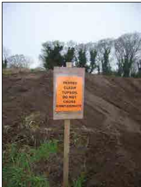
Photograph 14: Example of good stockpile management with warning signs to demonstrate areas of inert topsoil.
