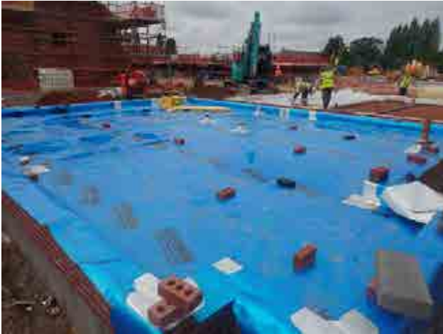
Photograph 2 and 3: Check general condition of gas membranes with photographs showing the plot in context.
