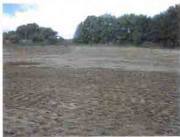
On-going re-compaction of materials in LRDM (July – October 2007)
