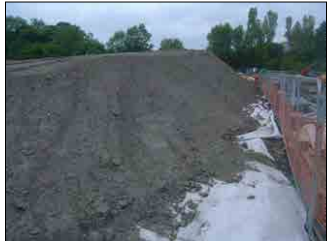
Photograph 13: Example of good stockpile management with soils placed on geotextile with fences to prevent accidental cross-mixing.
