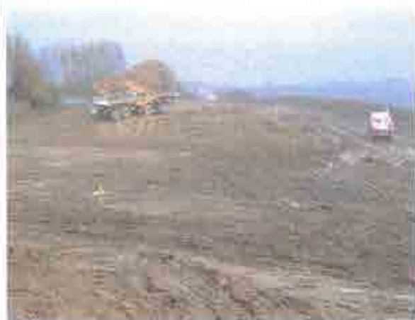
Excavation of lagoon area (November 2003)
