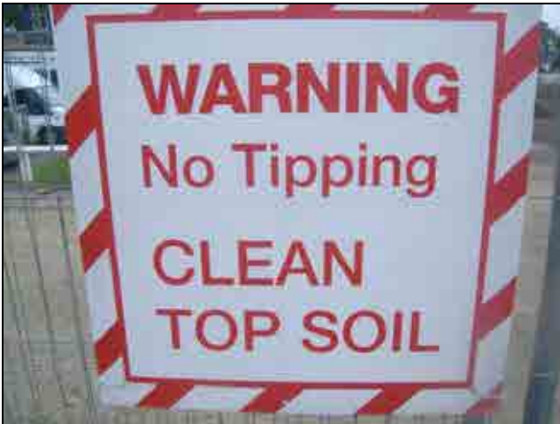
Photograph 12: Example of good stockpile management with warning signs to demonstrate areas of inert topsoil.
