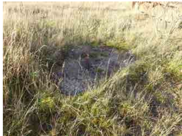
Photograph 4: Concrete pad with metal bar protruding left over from settlement monitoring.
