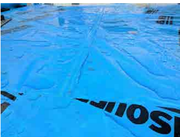
Photograph 6 and 7: Check >150mm overlaps of membranes and proprietary tapes placed and sealed or heat welded jointing with photographs taken.
