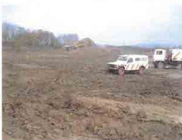
Excavation of lagoon area (November 2003)
