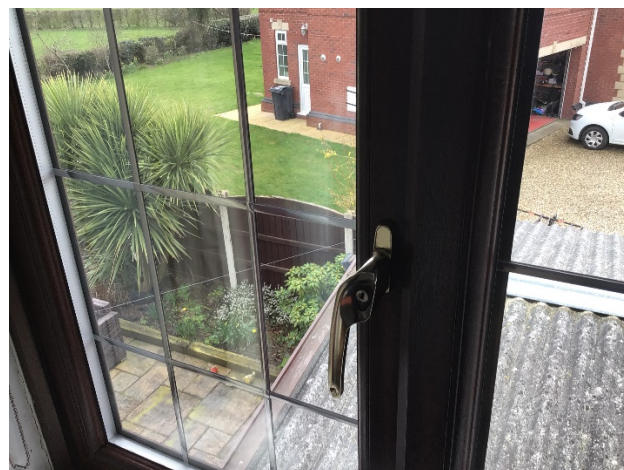
Photograph 2 view from bedroom
