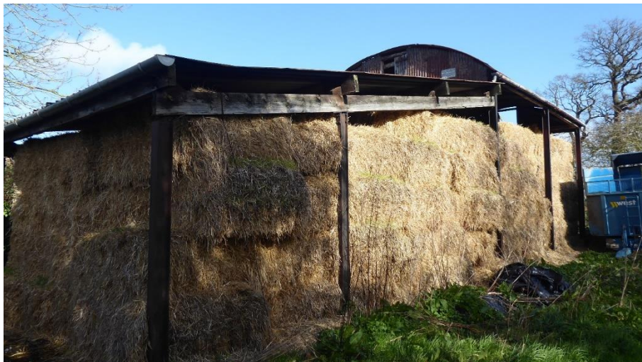
Figure 4.6 View of building 2 from south
