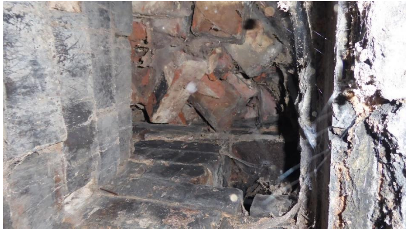
Figure 4.21 Blocked chimney
