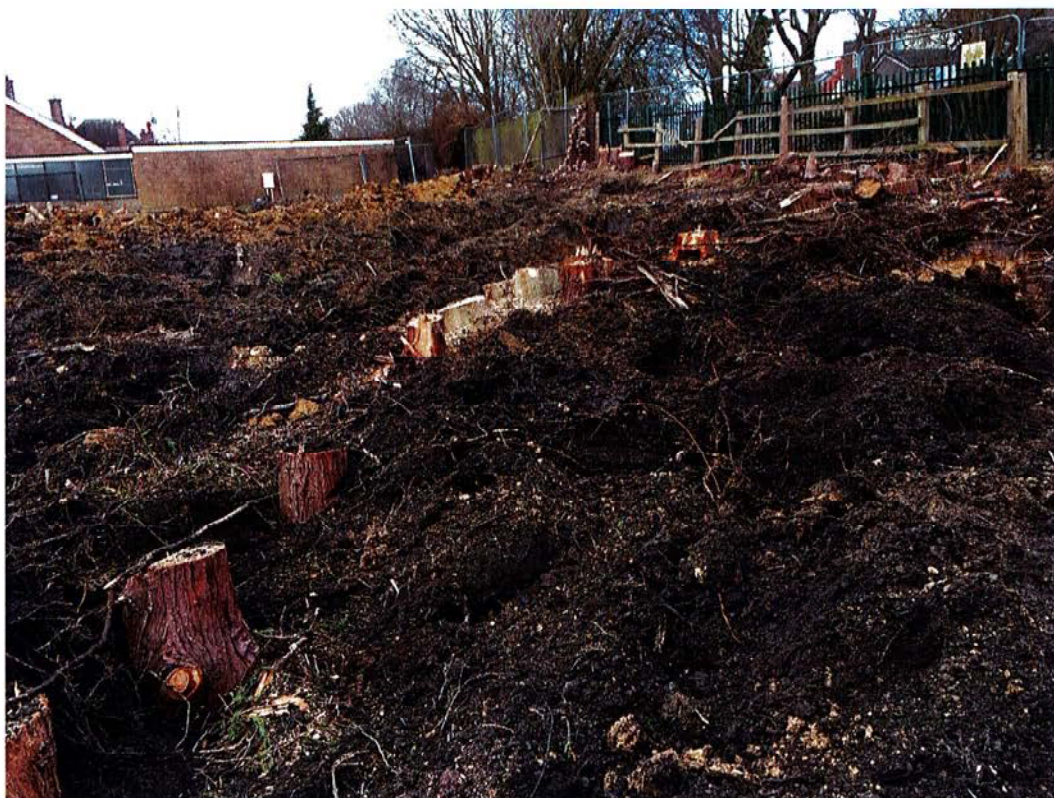
Photograph 3 looking north post demolition
