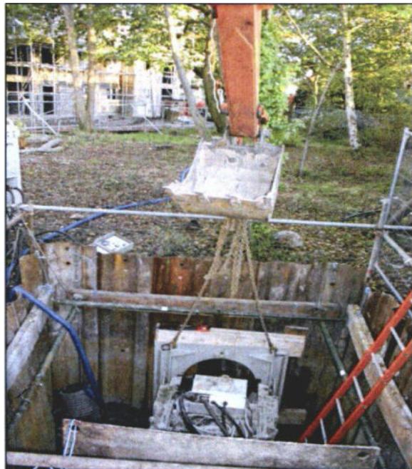
Photo 44: If possible, thrust boring is the preferred option for installing service routes through the RPAs of important trees, but there has to be space at the start and finish to dig substantial working pits.
