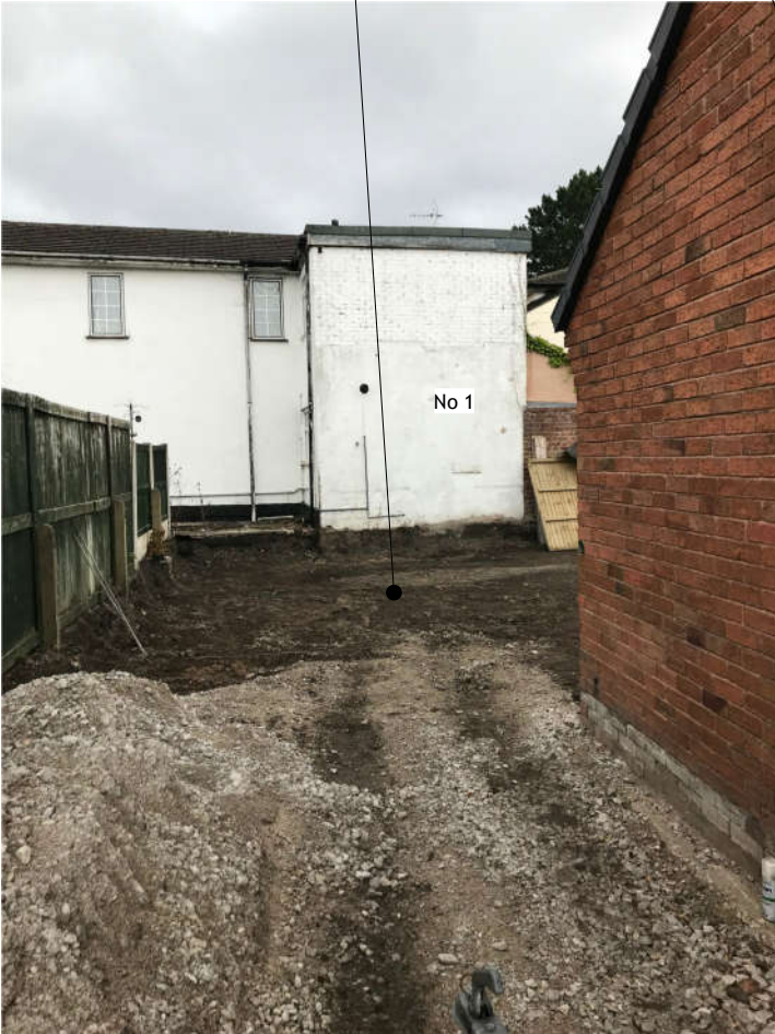
VIEW FROM EXISTING DRIVEWAY (EAST)
