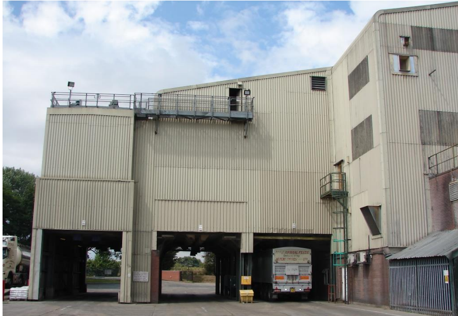
That part of the existing building ( Target Note 16a ) to which the proposed finished product storage/ out-loading facility would be attached.
