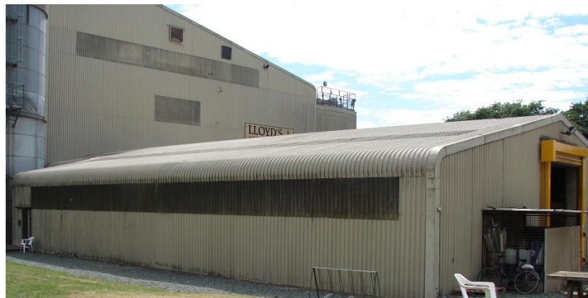
That part of the existing building ( Target Note 16 ) closest to the location of the proposed extension.
