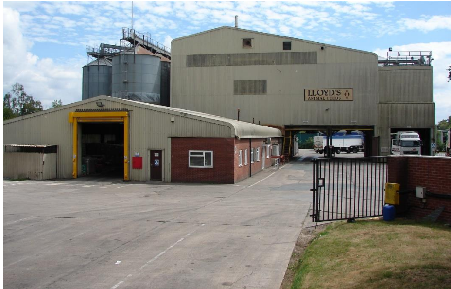
The building at Target Note 16 on the left foreground with the main industrial unit in the background ( Target Note 16a ).
