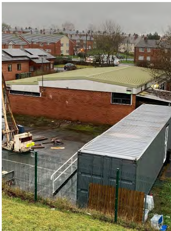
Photo Ref 10: Site overview looking south, showing roof of existing building
