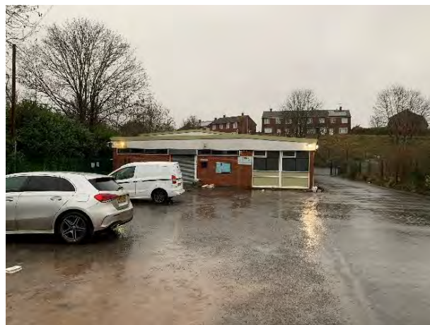
Photo Ref 2: View to southern elevation of existing building
