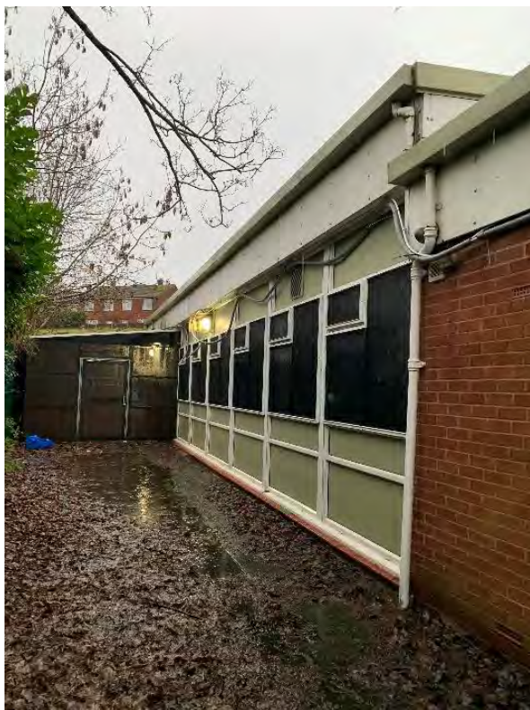
Photo Ref 9: Building western elevation
