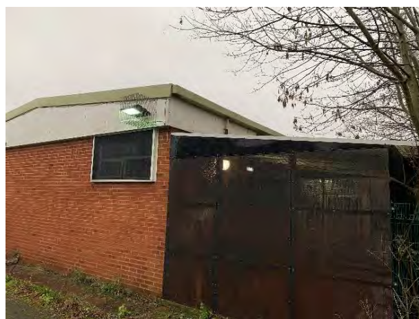
Photo Ref 4: Northern elevation of existing building
