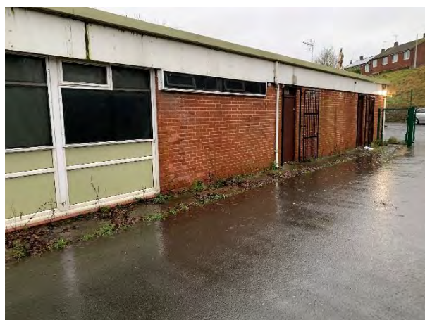
Photo Ref 3: Eastern elevation of existing building
