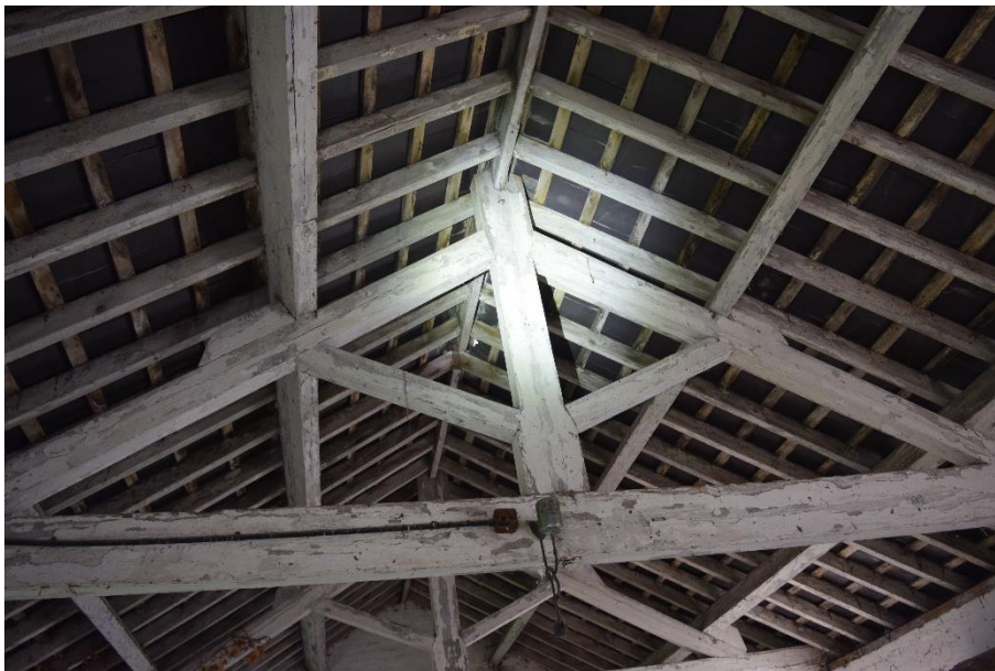
Figure 4.3 Roof space of building 1
