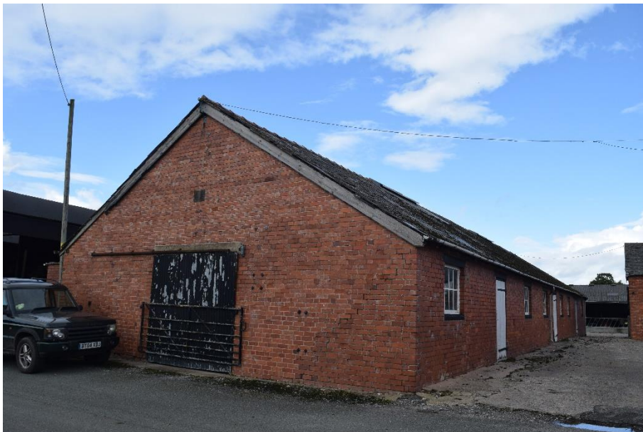
Figure 4.7 External view of building 2 from south
