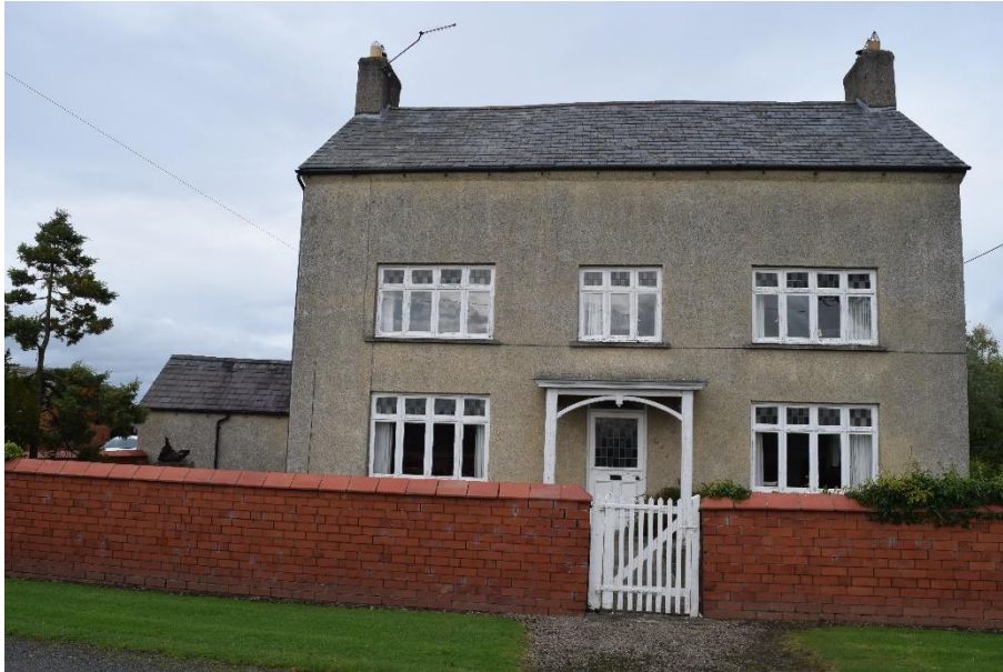
Figure 4.20 Farmhouse to east
