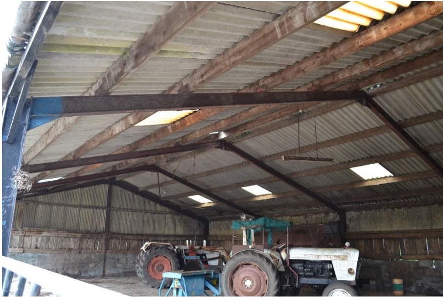
Figure 4.16 Interior of building 4
