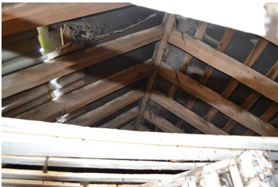
Figure 4.12 Roof space of building 3
