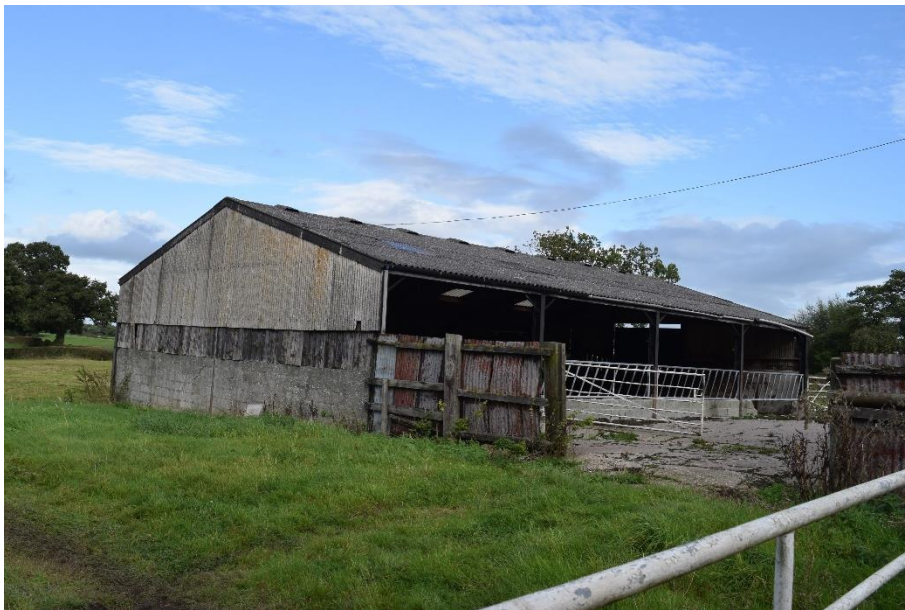
Figure 4.15 External view of building 4 from southwest
