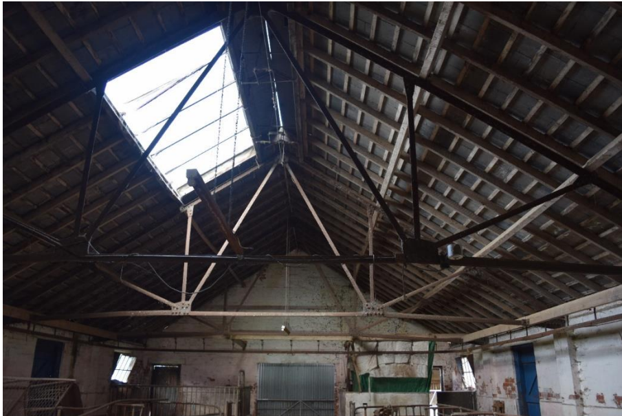
Figure 4.8 Roof space of building 2
