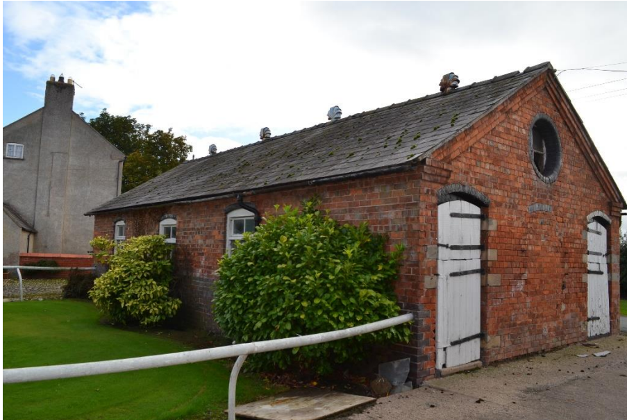
Figure 4.2 External view of building 1 from northwest
