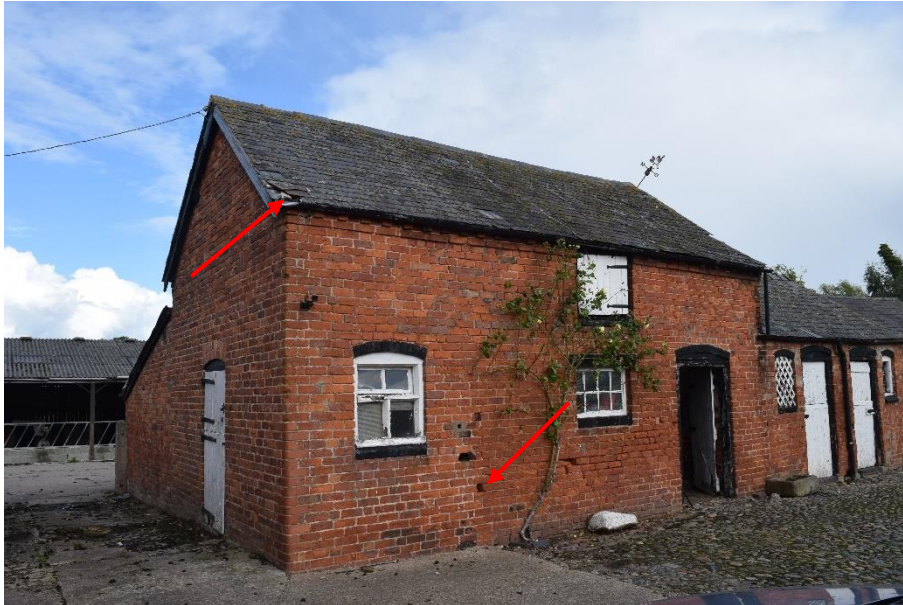
Figure 4.10 External view of front of building 3 from southwest with potential access points
