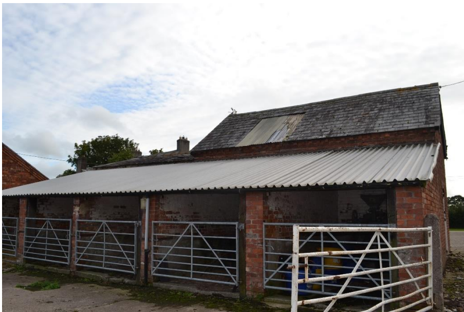
Figure 4.11 External view of building 3 from north
