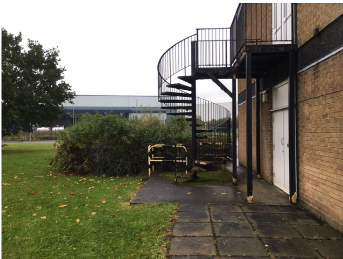
P13 – Corner of broadleaf shrub bed requires pruning to facilitate demolition and fence installation
