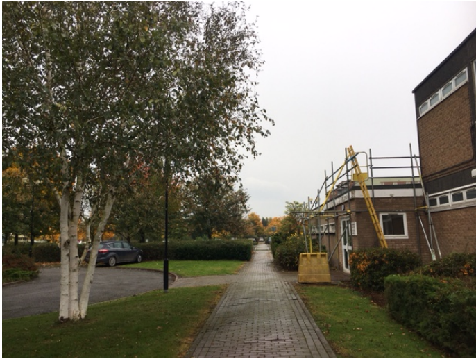
P1 – T2 crown low over demolition area contained within footpath (pruning specified)
