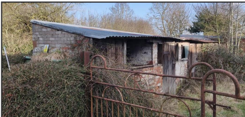
Photograph 4: showing most westerly compartment of Building 3
