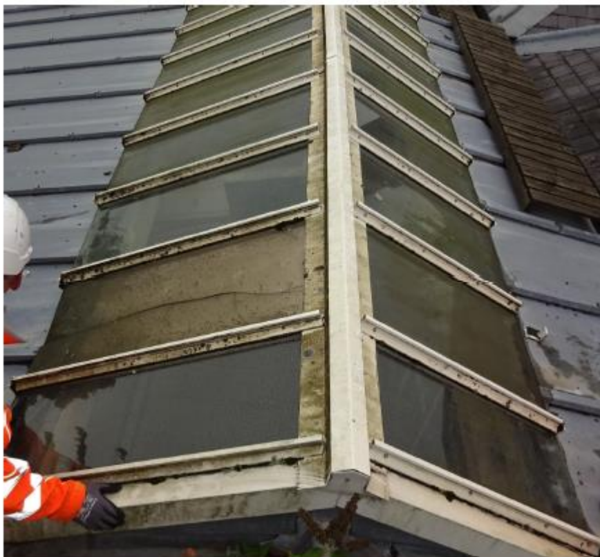
Picture 1 – Glazing Panels above platform 1 – Note aluminum glazing bar system
