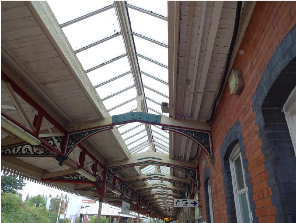
Photo 3 Underside of Platform 1
