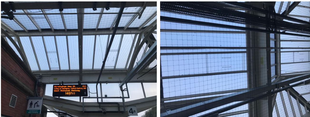
Photo example- 6 Shrewsbury Station, Shropshire with access hatches installed
