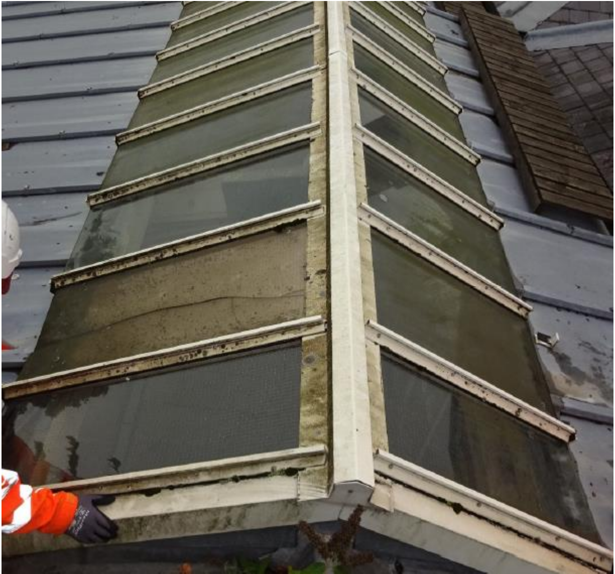
Figure 2: Glazing Panels above Platform 1 – showing aluminium glazing bar system used
