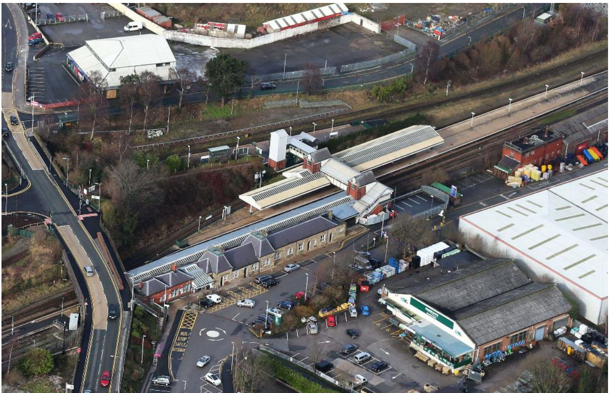
Figure 1: Aerial View of Wrexham General Railway Station
