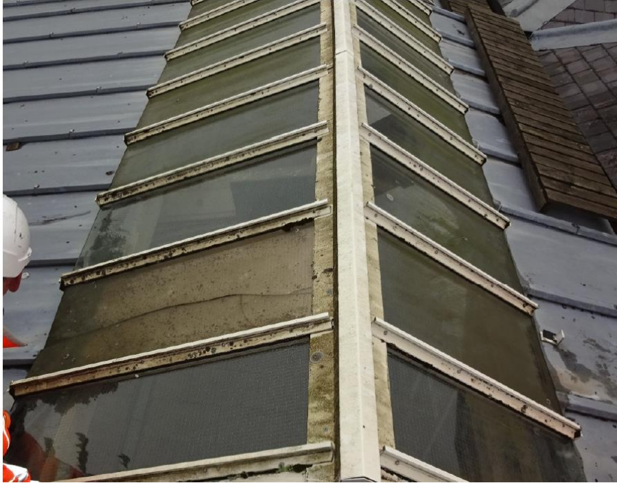
Photo 1 Glazing on Platform 1 Note aluminium glazing bars
