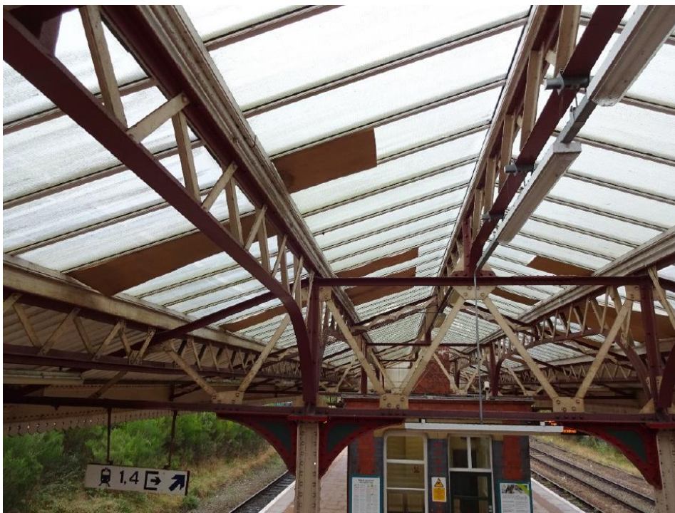
Photo 4 Underside of platform 2&3
