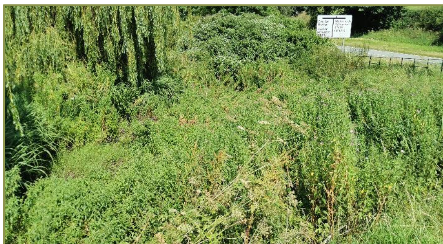
Figure 3.12: View of Hanmer Mere and Box Culvert to the north of the mere
