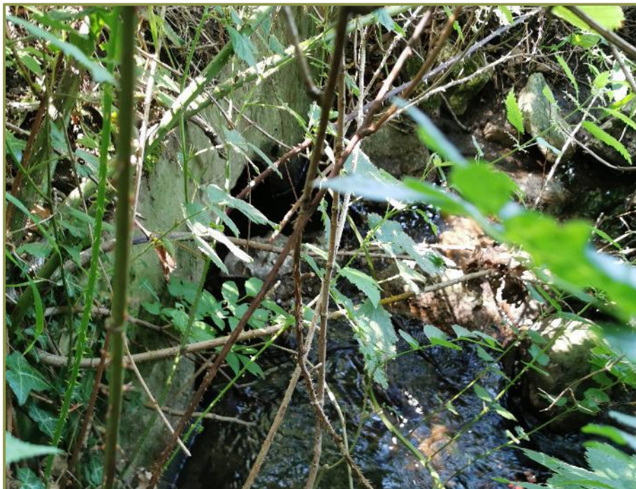
Figure 3.10: Ø600mm culvert conveying flow beneath A539.
