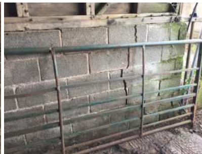
Collision Crack.
