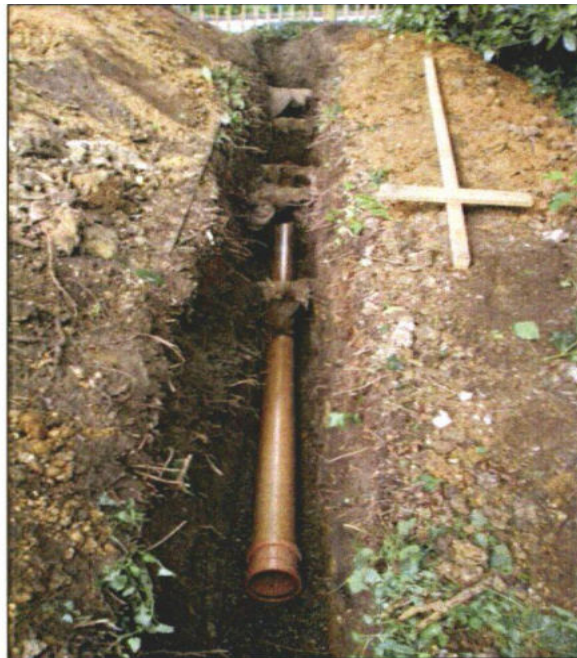
Photo 45: Continuous trenches dug by hand so that important roots can be retained (with the service ducting threaded beneath) is an effective means of minimising damage (note the ground protection boards with soil piled on top on the left).
