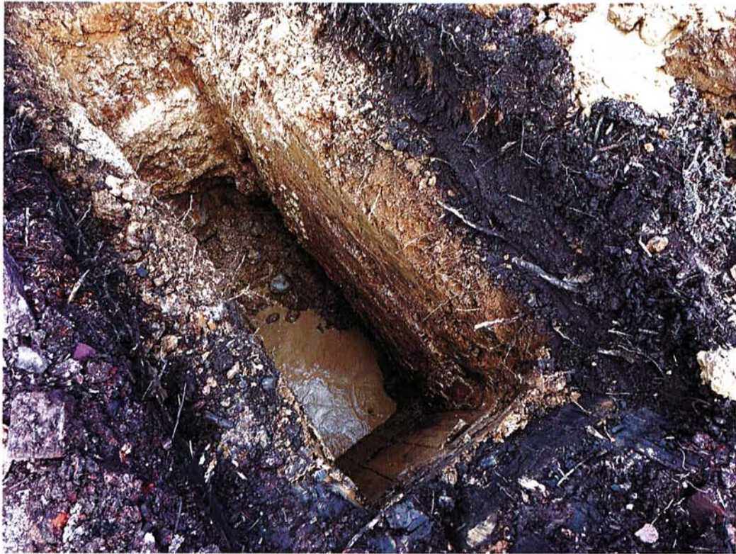
Trial Pit 07 – Pit walls
