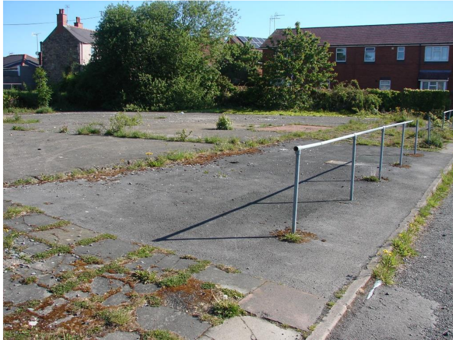
The footprint of a demolished building in the north of the survey site.
