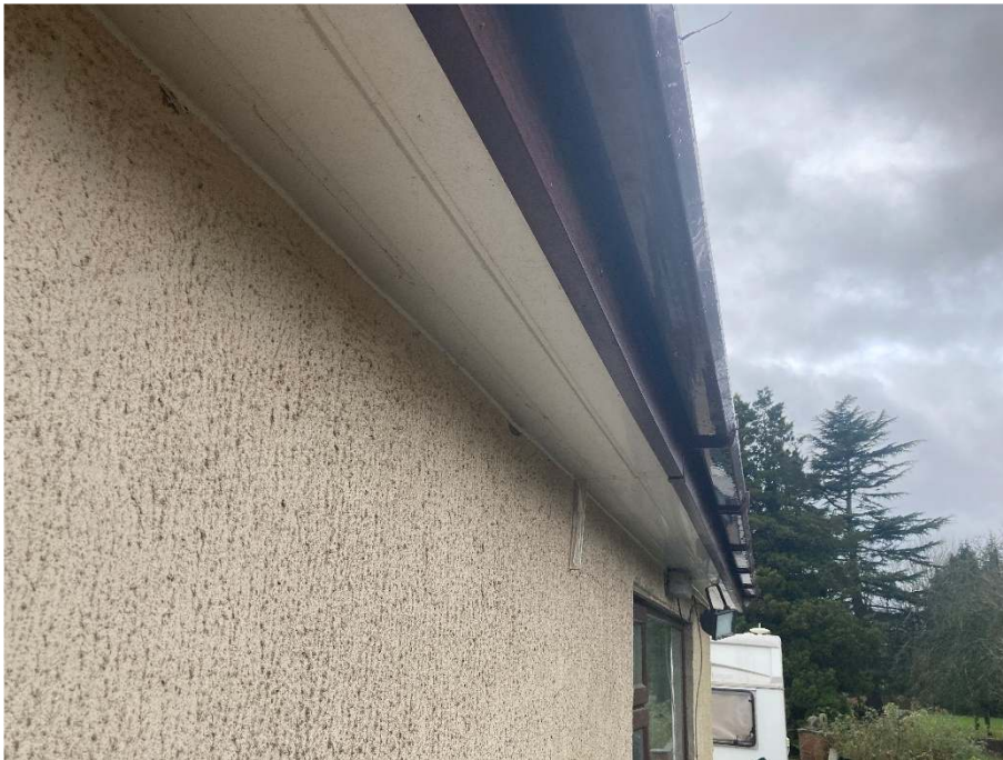
A1.5 Plate 5: Soffit box on northern and southern aspects well sealed no gaps for bats
