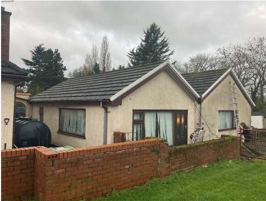
A1.3 Plate 3: View of eastern (back) and southern aspect of the garage
