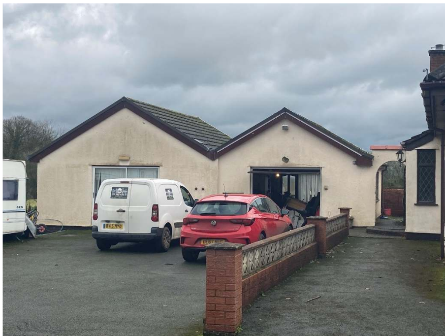
A1.1 Plate 1: View of front and western aspect of the garage
