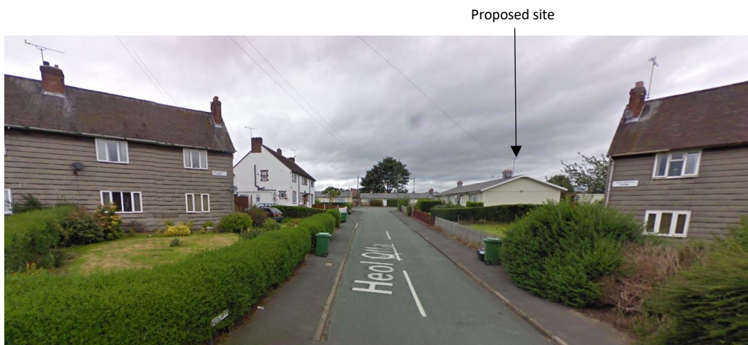
View of plot 83&85 from Heol Kenyon (Prefabricated bungalows on the site have previously been demolished)
