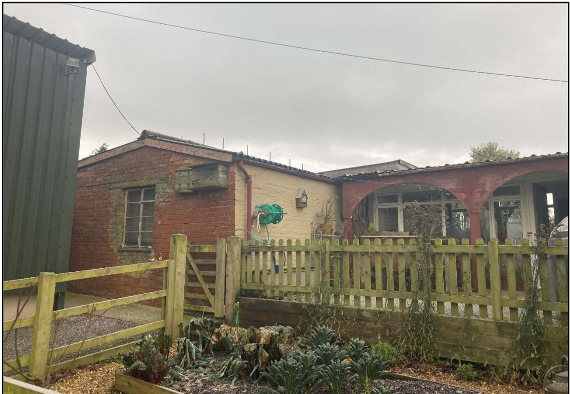
A1.2 Plate 2: View on eastern aspect of building
