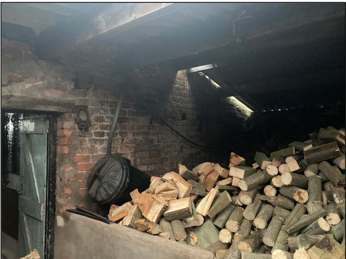
A1.4 Plate 4: Interior of structure with associated log pile
