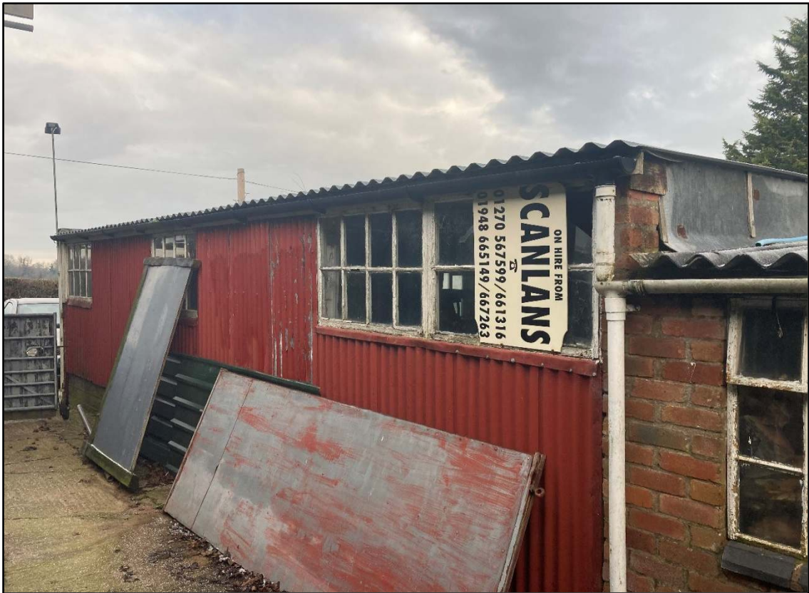
A1.3 Plate 3: View on southern aspect of building
