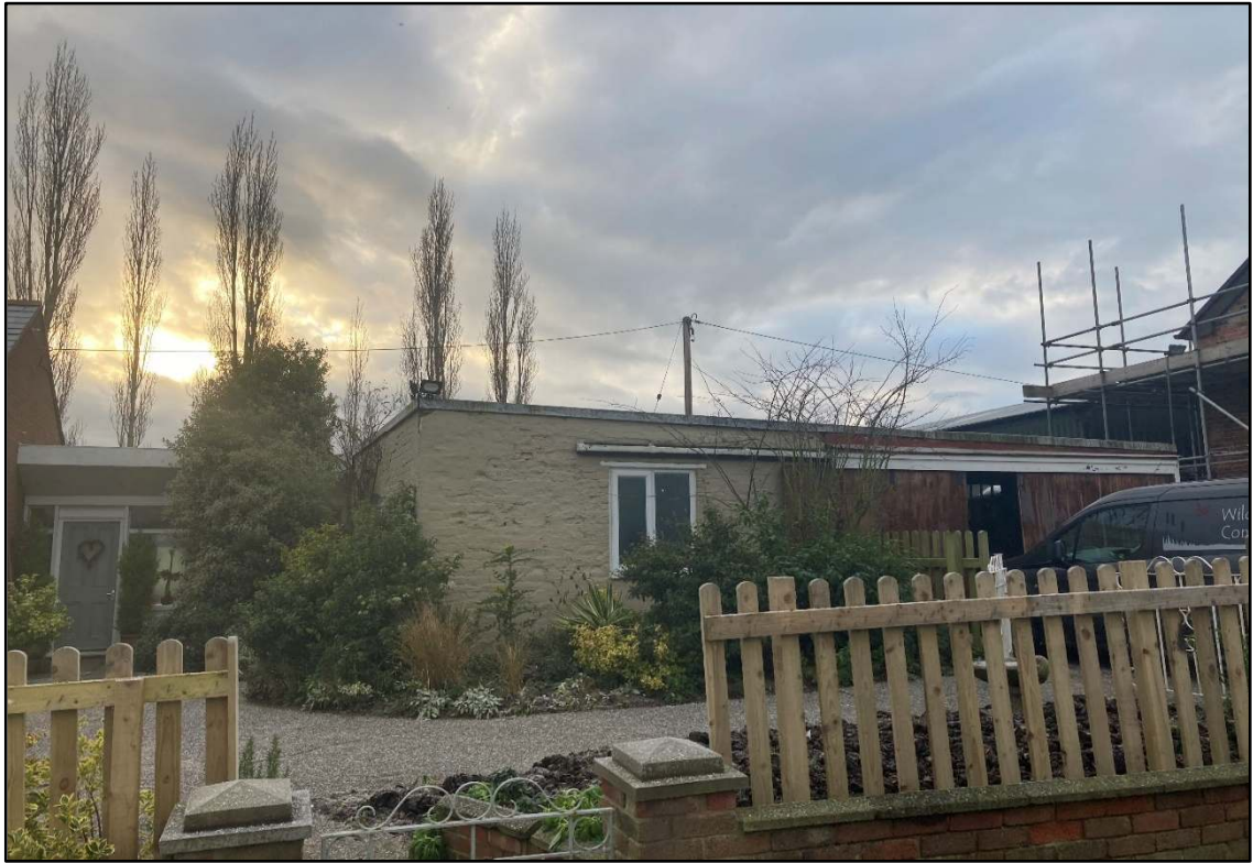
A1.1 Plate 1: View on western aspect of building
