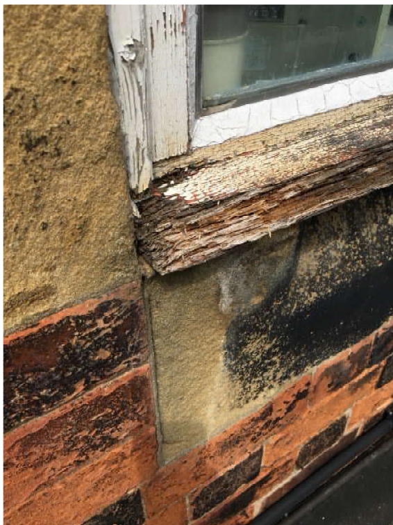
Figures 4 and 5 – rotting timber on the window frames to the extension and to the kitchen
