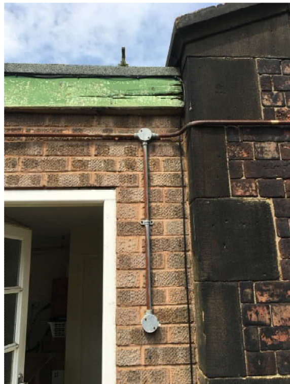
Figures 6 and 7 – green pipework and green soffits with evidence of rotting and warping.
