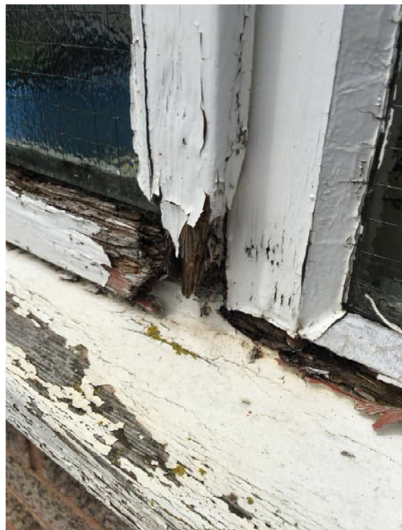
Figures 4 and 5 – rotting timber on the window frames to the extension and to the kitchen
