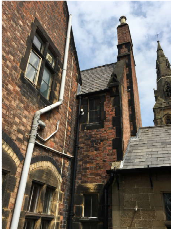
Figure 3 – the existing adjacent windows, showing the stone mullions
