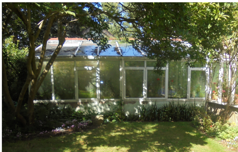
Existing Conservatory which is to be demolished
