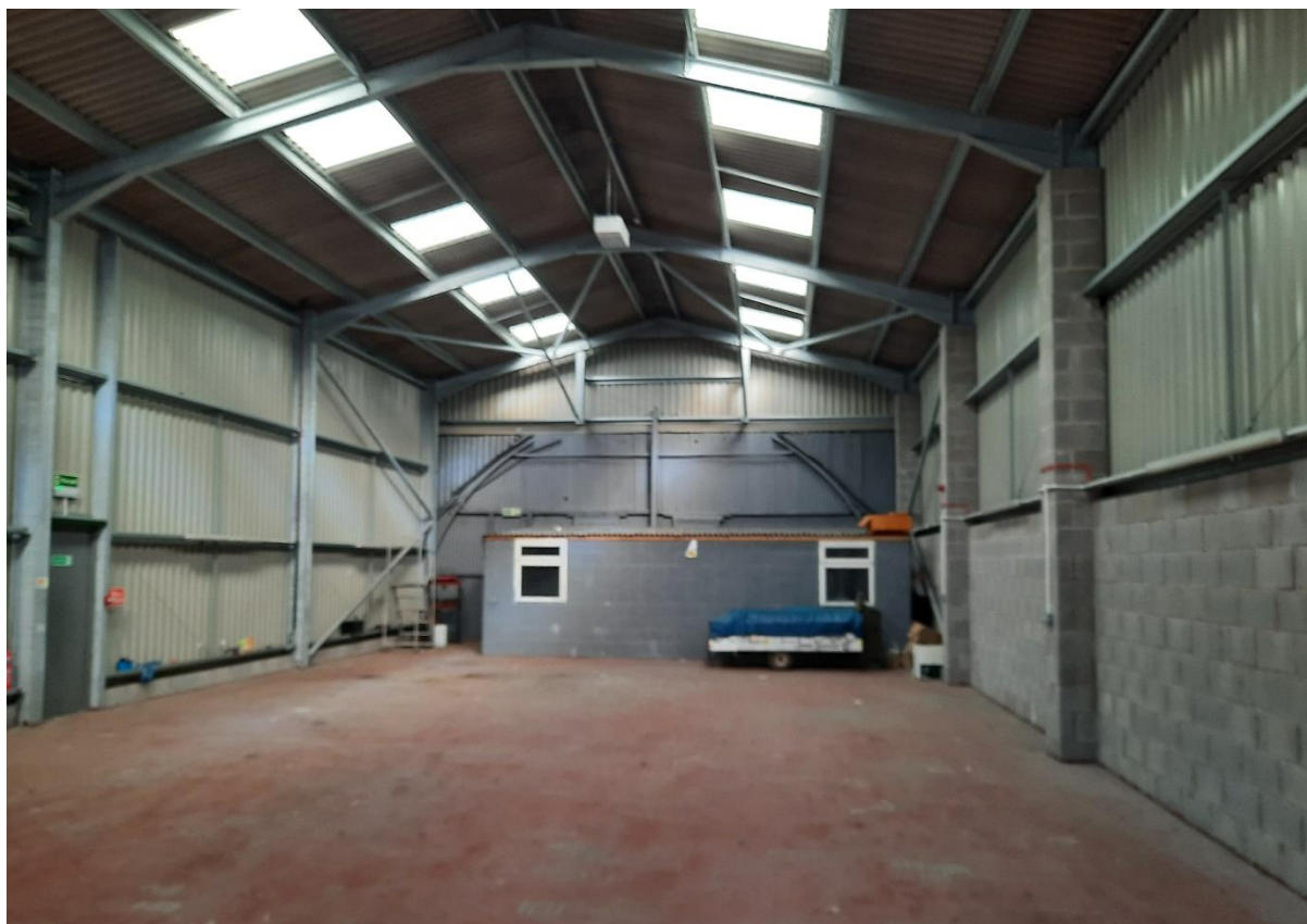
Figure 1 Phot showing internal of large central metal building.
